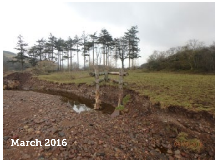
Figure 20 continued. (D) stabilisation of gravel deposited by the September 2012 flood event through vegetation colonisation and (E) erosion of floodplain and material surrounding the piles of a structure at Clifton caused by natural channel movement. Note the removal of two of the pile anchors presumably by the December 2015 or January 2016 floods (see Figure 19 for locations).
