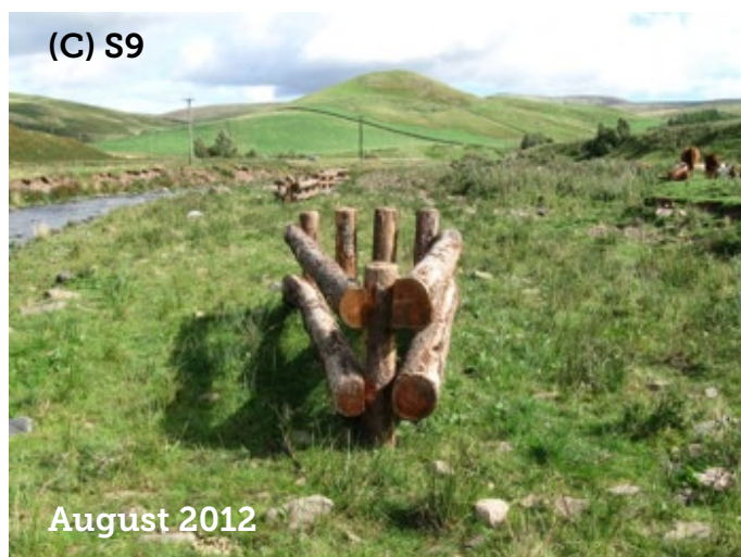
Figure 20: Selected examples of different responses at BAELJs (see Figure 19 for locations of structures). (A) deposition on the upstream side of a Kelsocleuch structure, (B) capture of debris and formation of scour pools at Bar 1, Swindon Haugh, (C) capture of debris and deposition of a gravel sheet upstream of a structure at Bar 2, Swindon Haugh (see Figure 19 for locations). Figure 20 continues overleaf.
