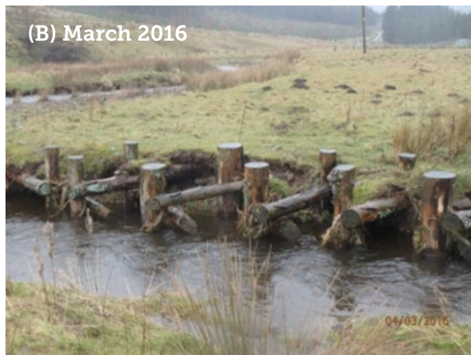
Figure 27: Downstream section of Structure 1 between August 2012 and March 2016. Note the erosion of placed gravel backfill and turf followed by progressive erosion of the bank.
