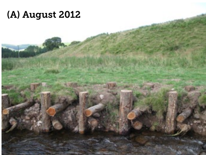
Figure 27: Downstream section of Structure 1 between August 2012 and March 2016. Note the erosion of placed gravel backfill and turf followed by progressive erosion of the bank.
