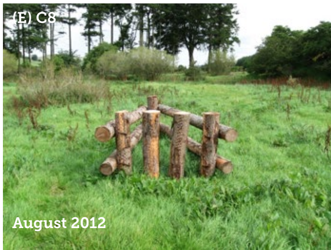
Figure 20 continued. (D) stabilisation of gravel deposited by the September 2012 flood event through vegetation colonisation and (E) erosion of floodplain and material surrounding the piles of a structure at Clifton caused by natural channel movement. Note the removal of two of the pile anchors presumably by the December 2015 or January 2016 floods (see Figure 19 for locations).
