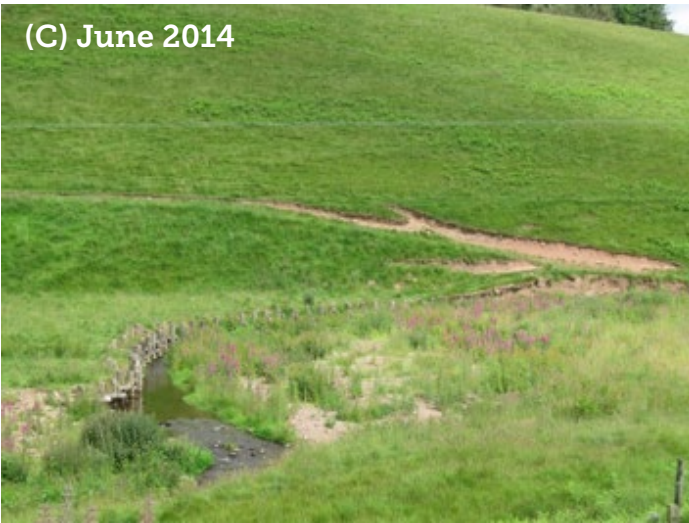
Figure 28: Changes to the channel and point gravel bar adjacent to Structure 1 between October 2012 and March 2016. Note narrowing of the wetted channel and the encroachment of vegetation over the stabilising bar.
