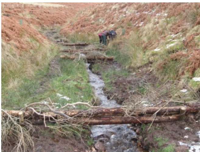
Figure 35: Flow restrictor S1 in the foreground photographed in February 2014 with structures S2 to S8 in the background. Note the gap (minimum of 0.3 m) below the timbers to facilitate fish passage.
