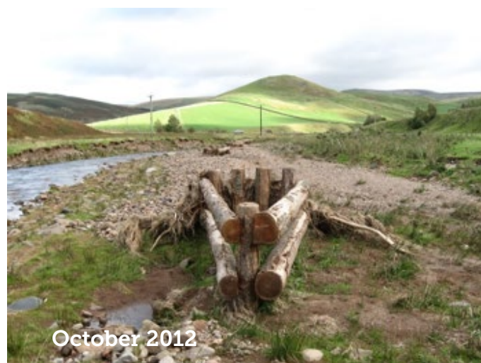
Figure 20: Selected examples of different responses at BAELJs (see Figure 19 for locations of structures). (A) deposition on the upstream side of a Kelsocleuch structure, (B) capture of debris and formation of scour pools at Bar 1, Swindon Haugh, (C) capture of debris and deposition of a gravel sheet upstream of a structure at Bar 2, Swindon Haugh (see Figure 19 for locations). Figure 20 continues overleaf.
