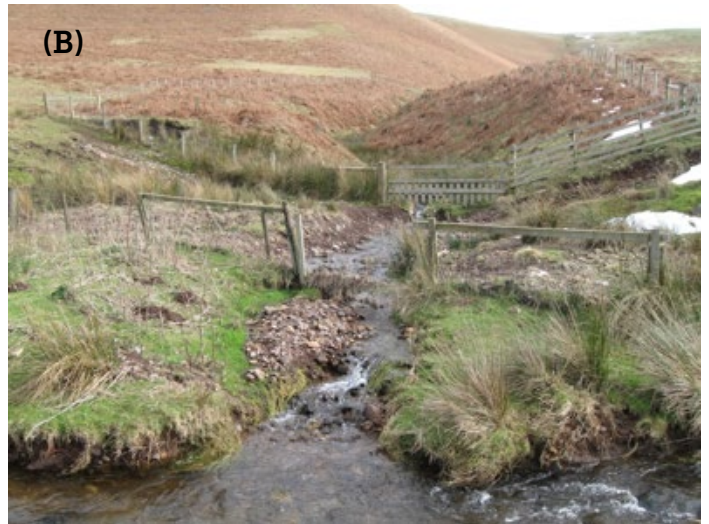
Figure 33: (A) Outlet of the Elm Sike in April 2013 before the flow restrictors were installed but with the fenced enclosure established. Note the large build up of coarse sediment in an alluvial fan between the fences. (B) The approximate same view in February 2016 after dredging of the channel in Autumn 2013 and following several flows sufficient to move coarse sediment and re-shape the channel (including 5th and 27th of January 2016 floods).
