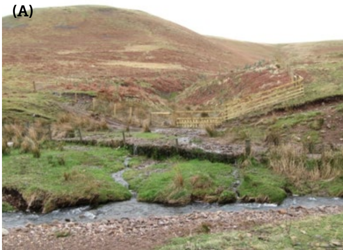
Figure 33: (A) Outlet of the Elm Sike in April 2013 before the flow restrictors were installed but with the fenced enclosure established. Note the large build up of coarse sediment in an alluvial fan between the fences. (B) The approximate same view in February 2016 after dredging of the channel in Autumn 2013 and following several flows sufficient to move coarse sediment and re-shape the channel (including 5th and 27th of January 2016 floods).
