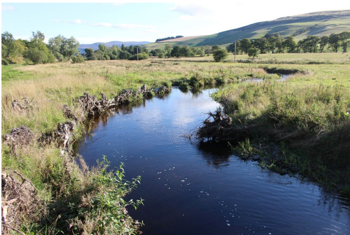
Newly completed meanders at Nether Kidston, showing root wads used to stabilise the banksides and create instream habitat
