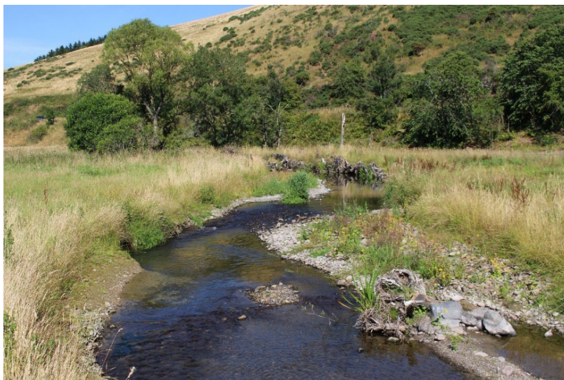
New channel form and placement of woody structures in newly created meander at Nether Kidston
