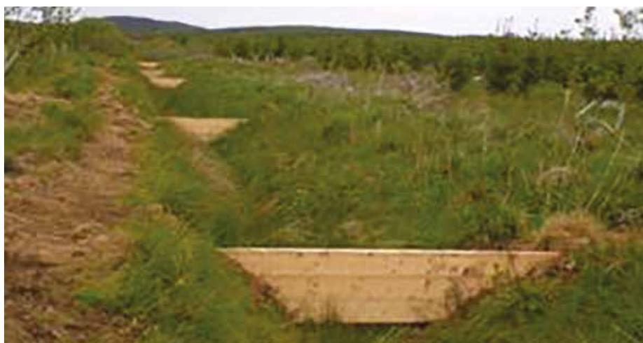
Figure 2.18. Small wooden ditch structures used to slow flows and encourage settling out of sediment in ditches in the Belford catchment, Northumberland (© Newcastle University).
