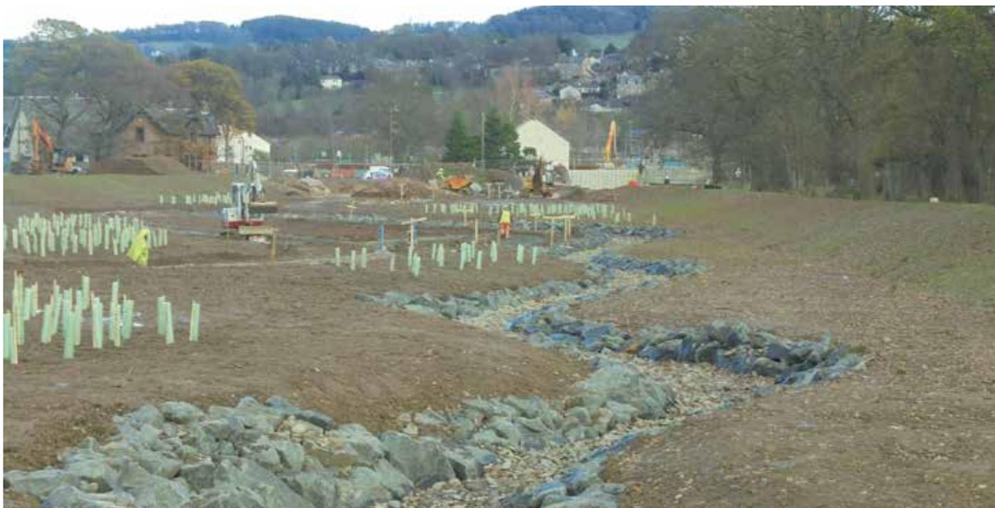
Figure 8.2. Realignment works on the Long Philip Burn, Ettrick Water (Tweed): These works form part of a wider suite of NFM and flood protection scheme measures implemented to help protect the town of Selkirk. The work and compensation to land managers was funded by the local authority's capital grant, Scottish Government and the Scottish Rural Development Programme (© Selkirk Flood Protection Scheme).
