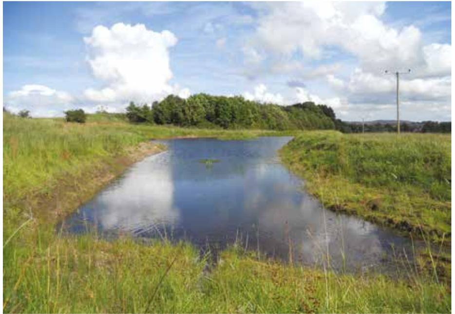
Figure 2.31. An offline storage pond in the Netherton Burn catchment, Northumberland: The pond has been designed in such a way as to offer additional water storage in times of high flow. The pond is supported by a series of sediment traps on the inflow points (© Tweed Forum).
