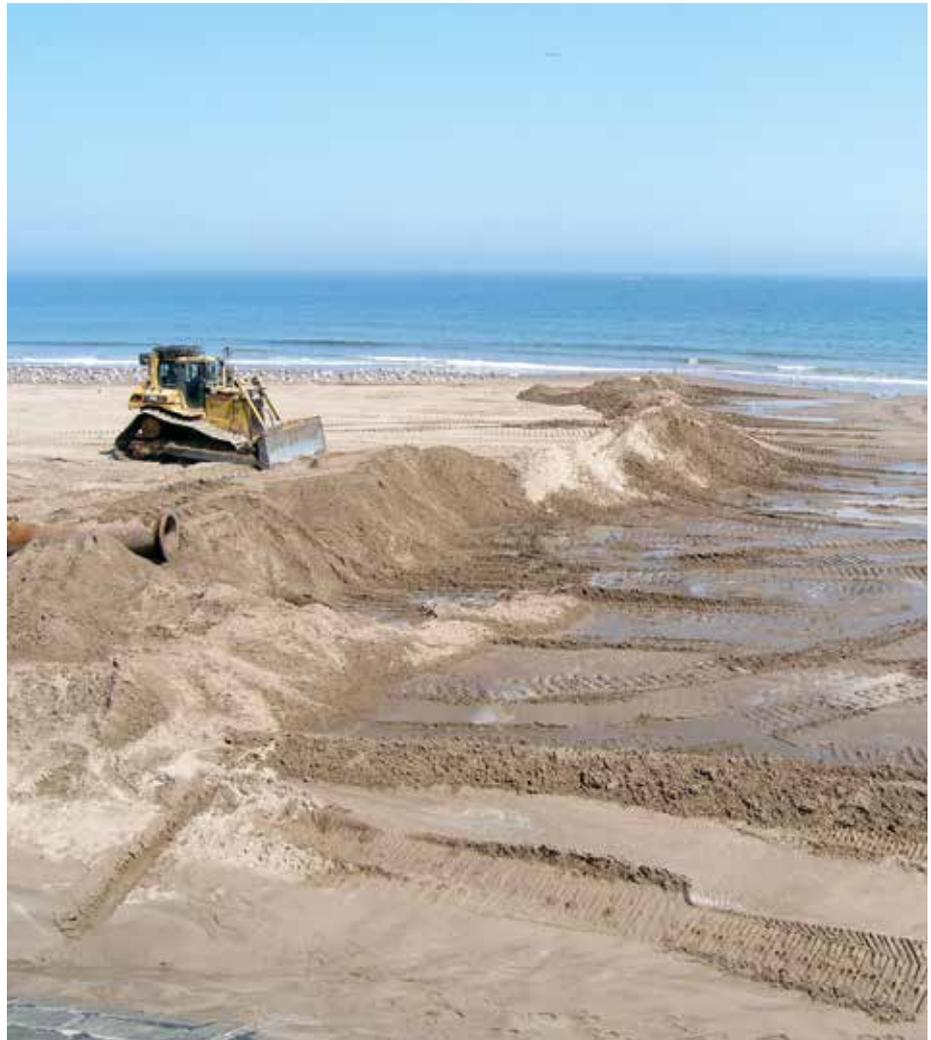
**Figure 3.20. Recharge underway at Aberdeen beach to protect sea defences and dissipate wave energy.**
