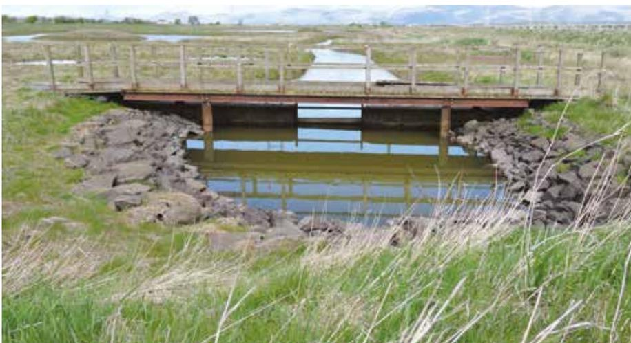
Figure 3.11. Regulated tidal exchange at Skinflats, Firth of Forth estuary: a pipe and sluice (pictured) mechanism was installed to regulate the inflow of sea water onto a grass field, providing a new line of defence and creating new habitat.
