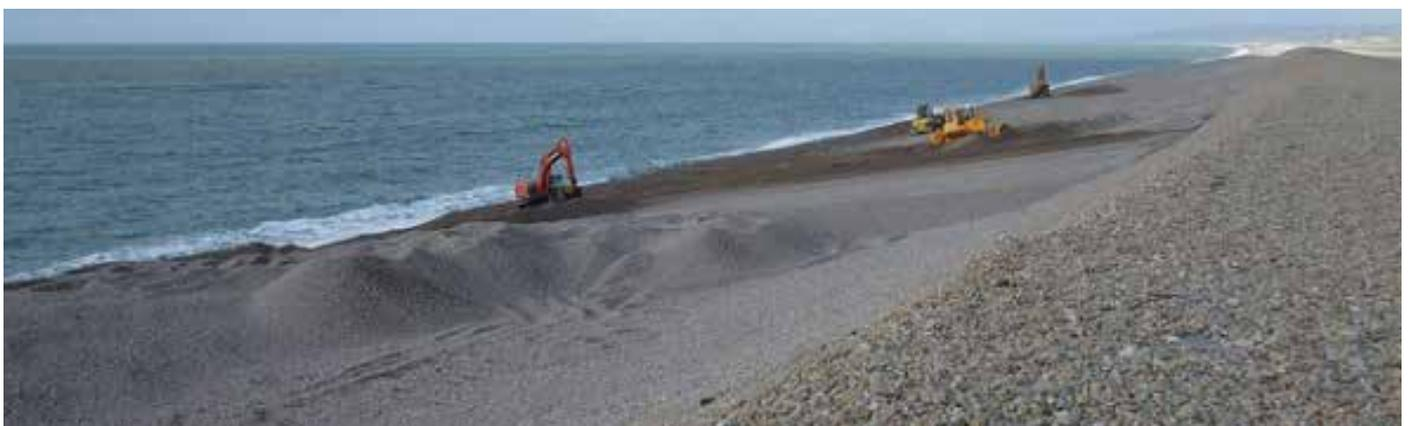
**Figure 3.18. Replenishment and reprofiling on the shingle at Chesil beach, Dorset: This work was undertaken in order to increase protection to the community of Chiswell following significant storms (© Environment Agency).**
