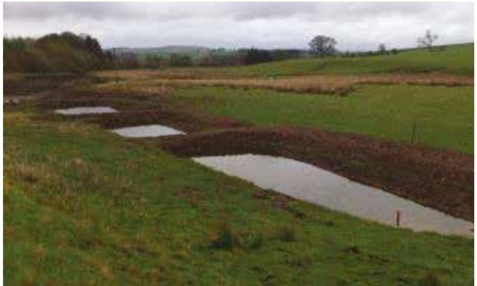
Figure 2.21. Three sediment traps constructed in series to intercept surface runoff and encourage settling out of sediment in the River Coquet catchment, Northumberland (© Nick Barber, Newcastle University).
