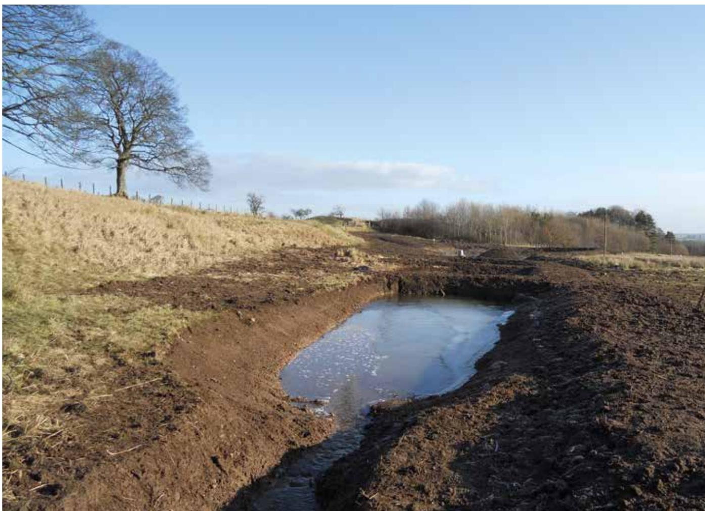
**Figure 2.22.** A series of sediment traps under construction in the Netherton Burn catchment, Northumberland. These sediment traps were constructed directly upstream of an offline storage pond in order to retain sediment and nutrients and slow the sedimentation rate in the main pond (© Tweed Forum).
