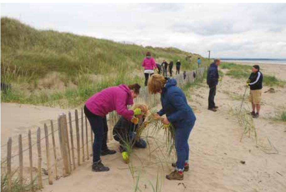
Figure 3.17. Sand dune restoration at St Andrews West Sands, Fife: Beach recharge, sand dune reprofiling and restoration was undertaken to improve the resilience of the dunes to manage flood and erosion risk (© R. Strachan/Fife Coast and Countryside Trust).
