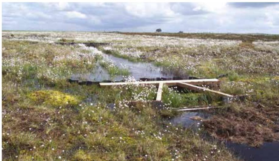
Figure 2.17. Restoration of blanket bog by blocking wide drains using plastic piling supported by timber frames at Blawhorn Moss, West Lothian.
