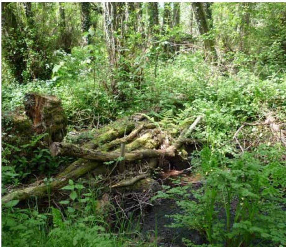
Figure 2.29. An in-stream structure in the Afon Gafenni catchment, South Wales: This structure is designed to slow high flows but does not impede fish passage. (© Forest Research).
